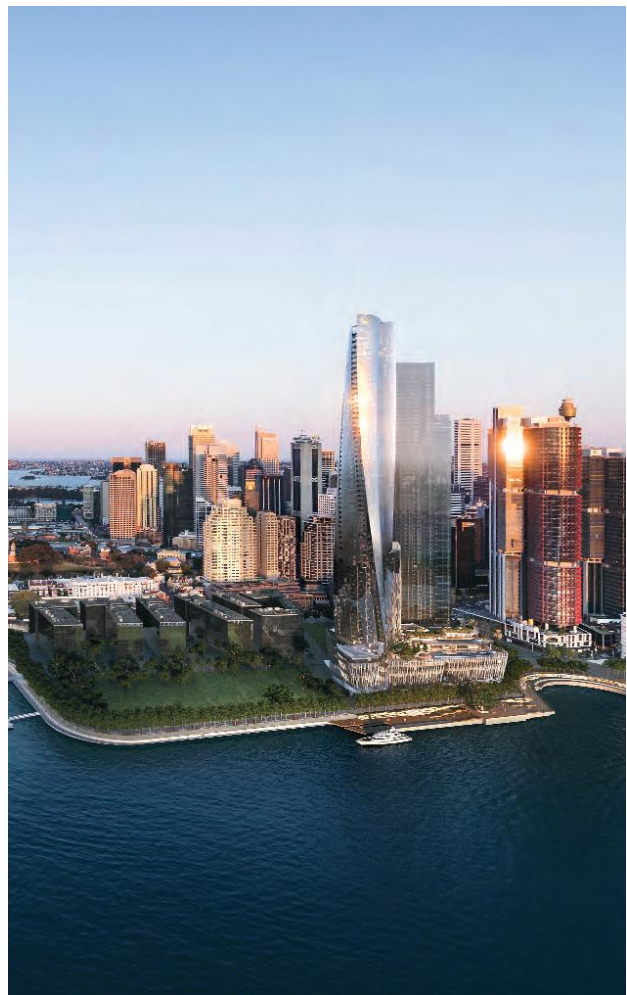
Large areas of public space have been created as part of One Barangaroo
