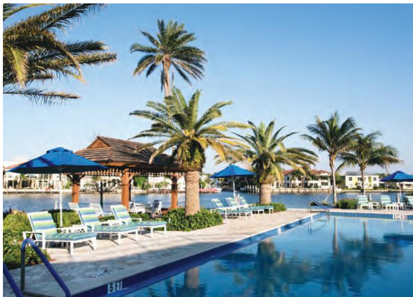
▶ Harbours Edge: senior living accommodation in Delray Beach, Florida.
